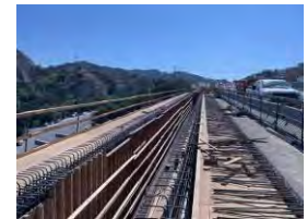
Gavin Canyon Bridge Right Formwork
