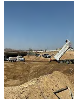
Embankment Fill at Rye Canyon
