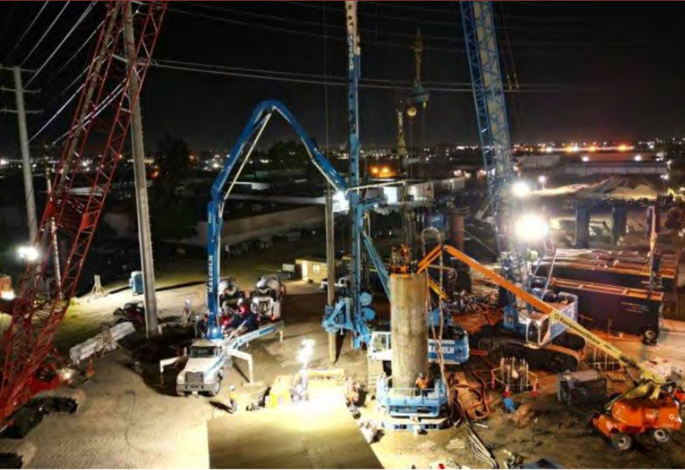
Caisson Installation
