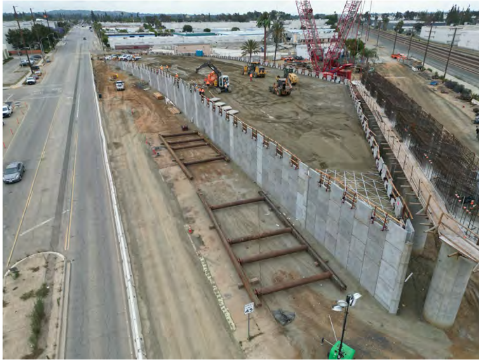
Mechanically Stabilized Earth (MSE) Wall No. 2
