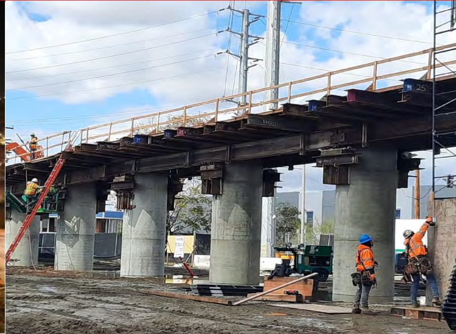
Bent Cap Construction
