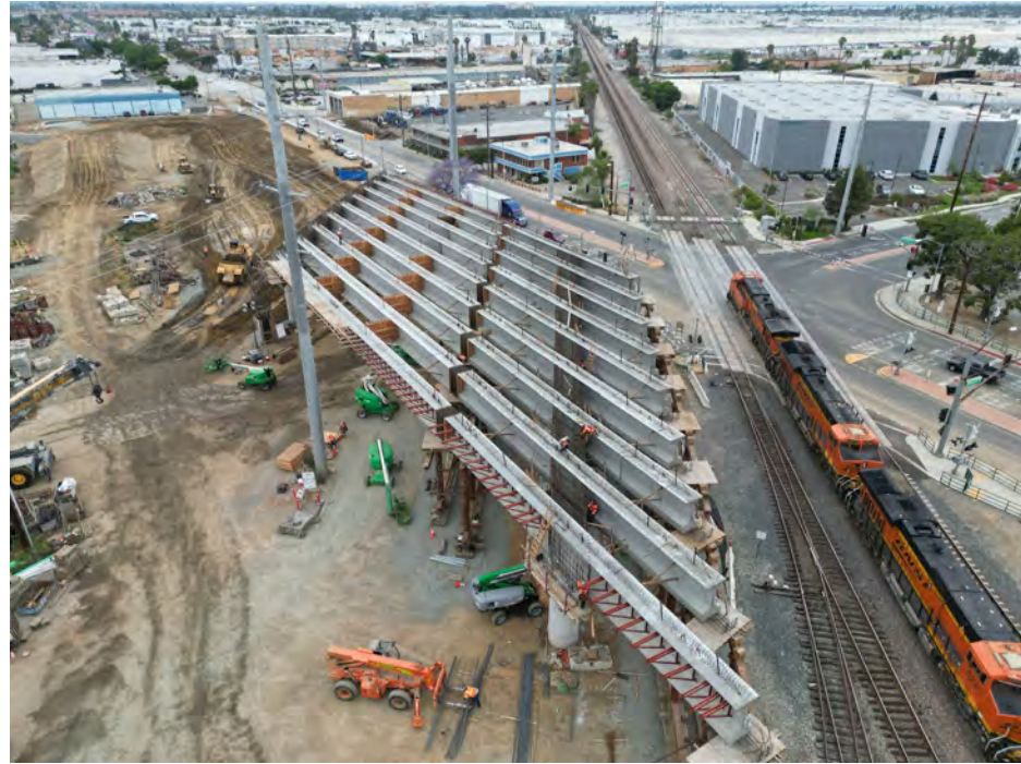
Precast Girders between Abutment 1 and 2
